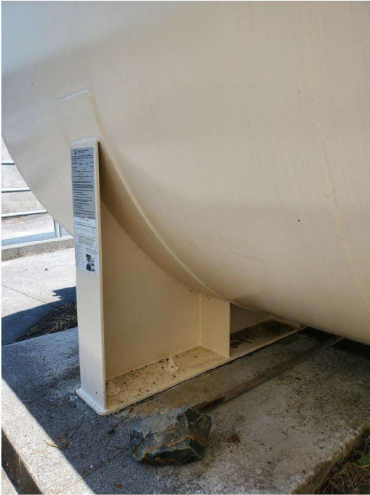
Photo 4. Foundation and Supports
