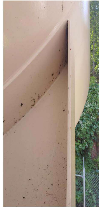
Photo 5. Foundation and Supports
