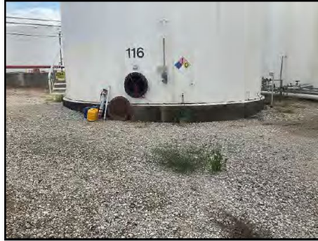
001 Grade Surrounding Tank Foundation
