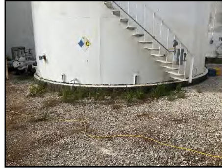
002 Grade Surrounding Tank Foundation
