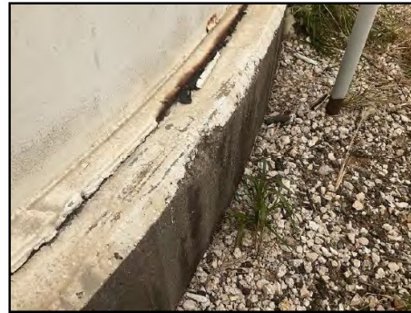
004 Spalling on Ringwall
