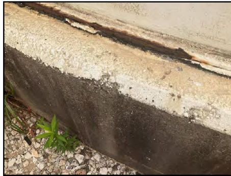
003 Spalling on Ringwall
