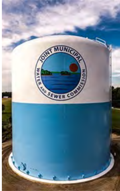
Field Erected Tank Section
