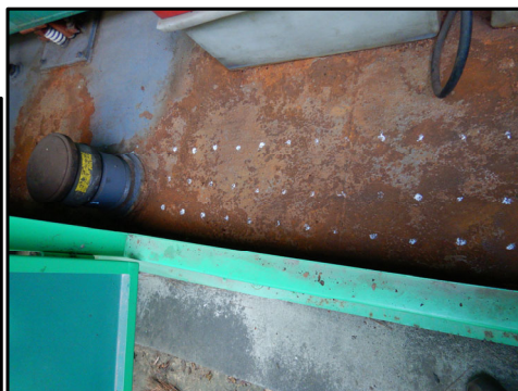
Tank top corrosion evaluated by UT inside the containment for generator
