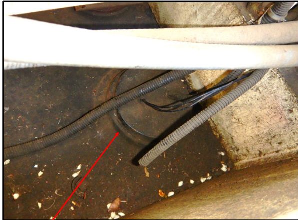
4-inch tank fitting on a base tank that should be location of emergency vent-but now used for sensors
