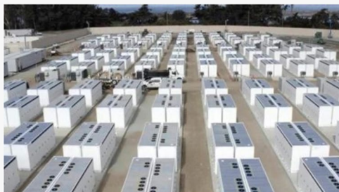
(This April 2021 drone image provided by Pacific Gas and Electric Company (PG&E) shows Tesla Megapack system in Moss Landing, Ca., that is now operational. (PG&E via AP).)
