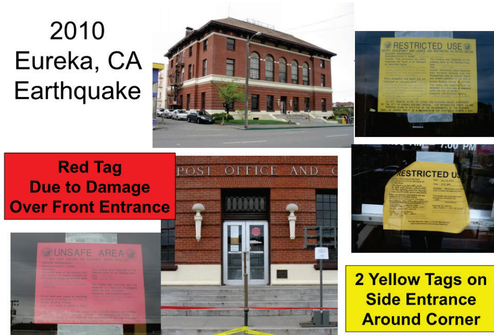
Figure 6-3 Placards posted on a government building in 2010 Eureka, California earthquake. Both yellow RESTRICTED USE and red UNSAFE placards were observed. Placards should be consistent on each side of the building.
