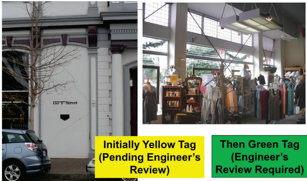
Figure 6-2 Placard posting approach in commercial building in 2010 Eureka, California earthquake. The initial placard was a yellow RESTRICTED USE tag with the recommendation for an engineering review. The placard was subsequently changed to a green INSPECTED tag, but still said an engineer review is required.
