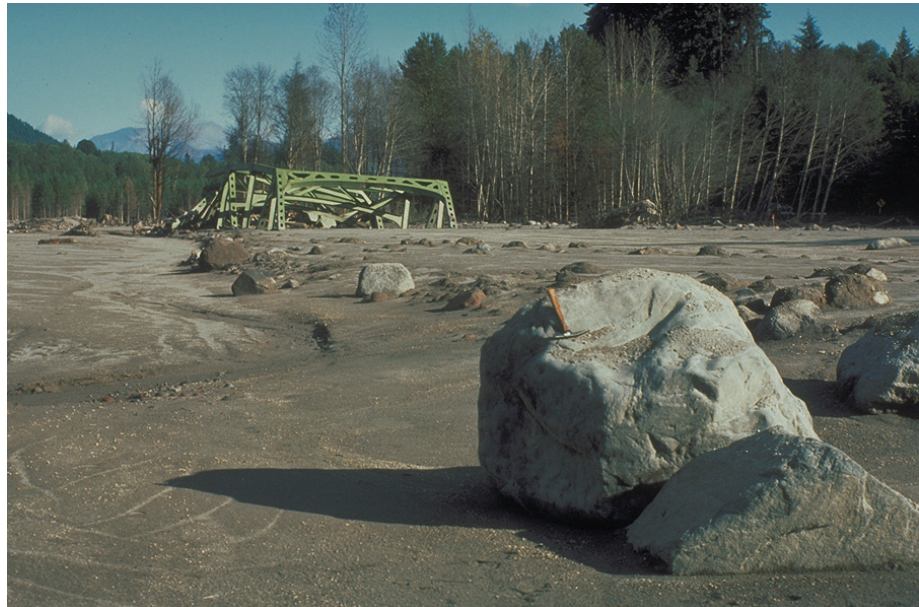
Figure 3-4 Bridge destroyed by lahar in North Fork Toutle River during eruption of Mount St. Helens, May 18,1980. Source: USGS https://volcanoes.usgs.gov/vhp/lahars.html
