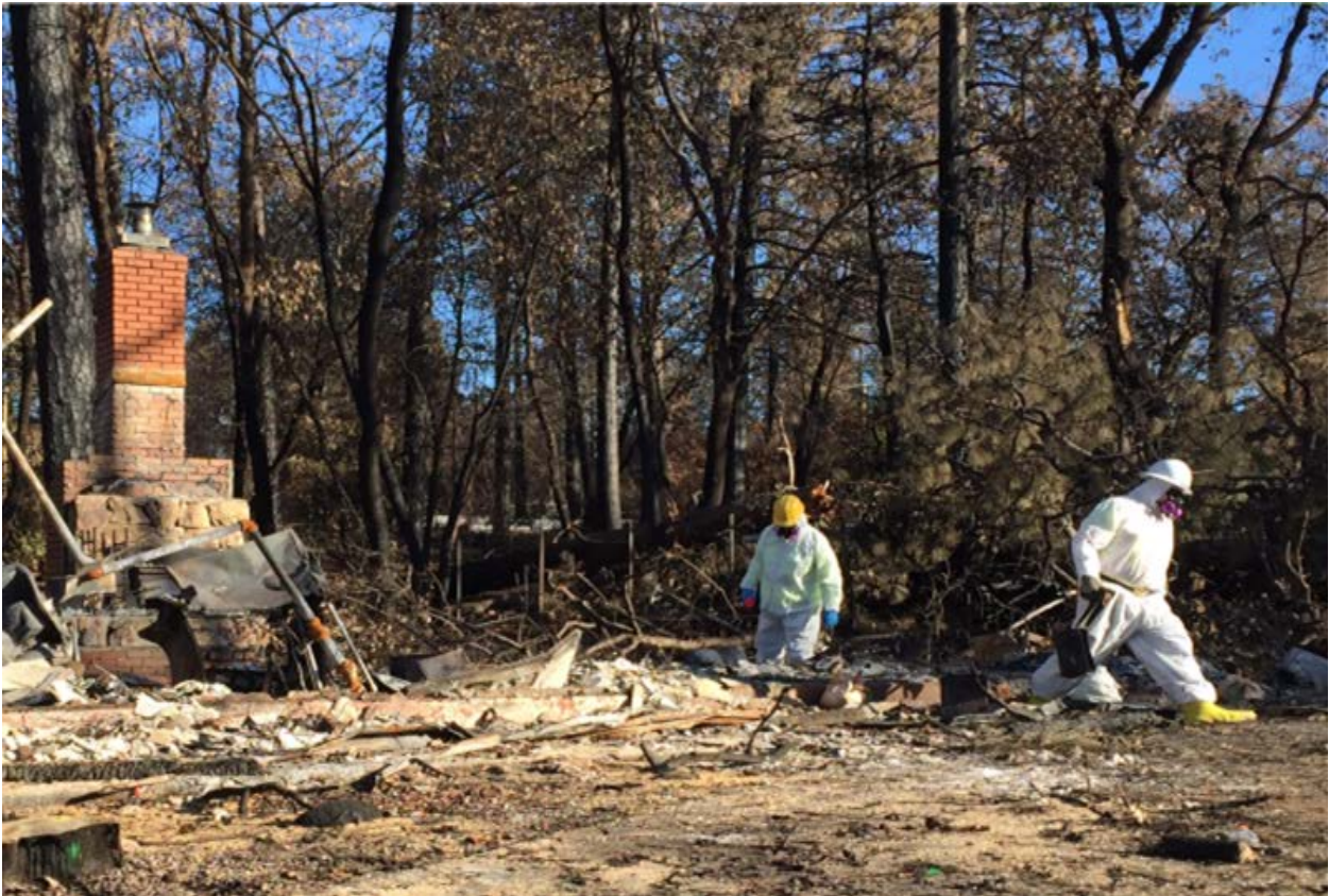
DTSC Haz Mat Crew evaluating structure with radiological monitoring instrument and a MultiRae Pro/Plus five gas meter or its equivalent.
